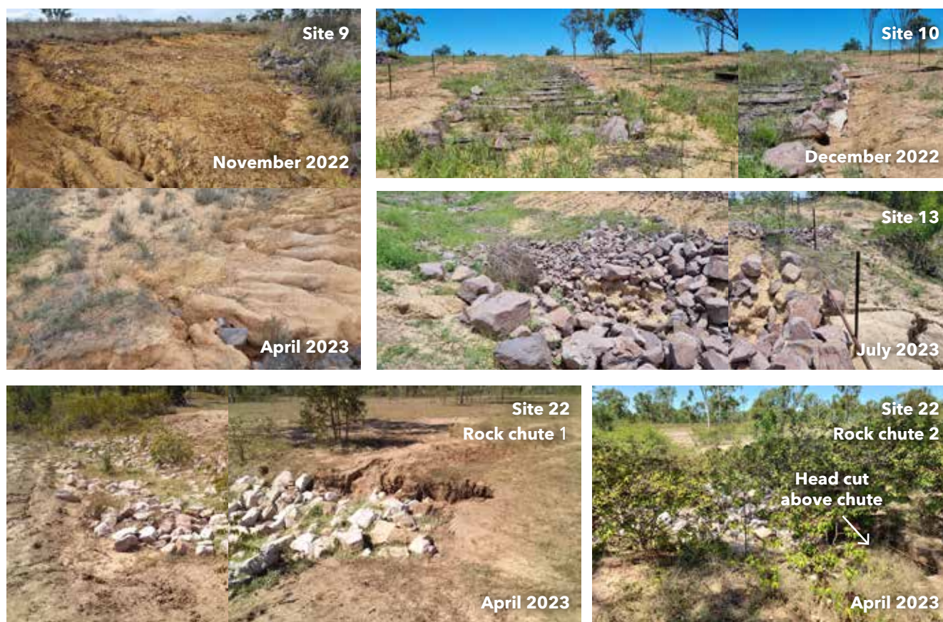
Figure 17. The five rock chutes at small-scale sites on highly erodible Sodosol soils. All have active erosion that will require continued maintenance to be effective.
