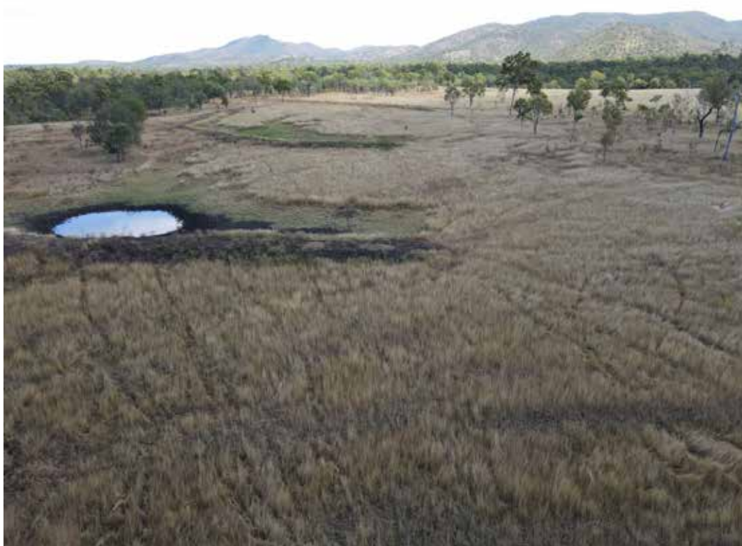
Figure 22. At Site 18 catchment work to control runoff into adjacent gullies involved a series of ‘rehydration’ banks. Photograph taken April 2024.
