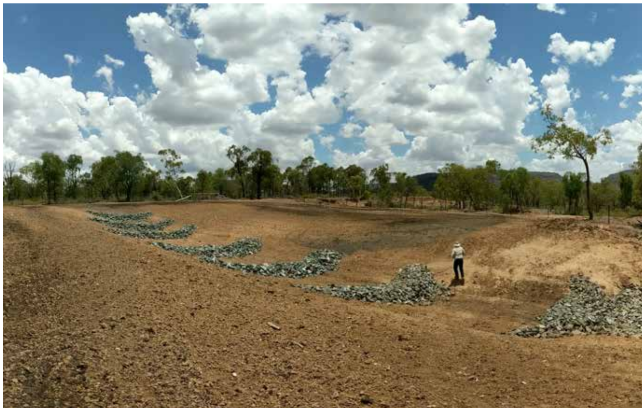
Figure 3. Porous check dams constructed with gabion-size rock on the large-scale Site 1 following the reshaping, ameliorants, seeding and fencing.
