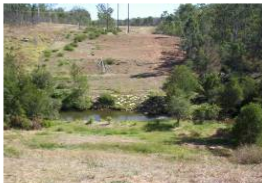
Plate 27: Rehabilitation of ROW across a watercourse
