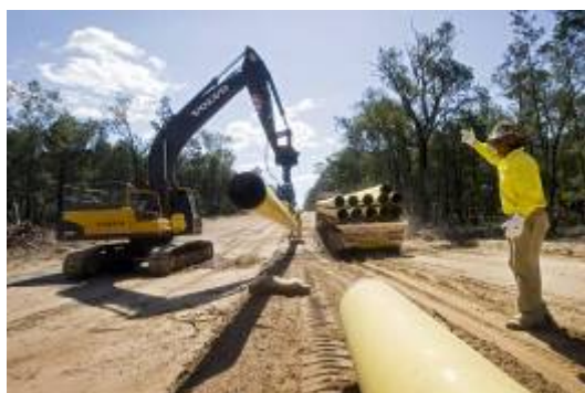
Plate 4: Pipeline stringing
