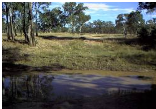
Plate 26: Rehabilitation of ROW across a watercourse
