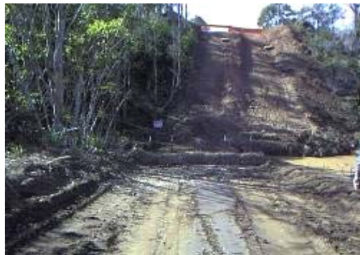
Plate 24: Open cut construction of watercourse crossing
