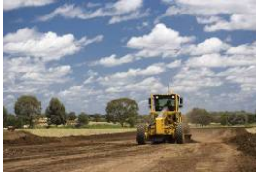
Plate 2: Typical grading of the ROW
