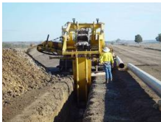
Plate 8: Trenching machine in operation
