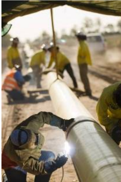
Plate 5: Pipeline welding
