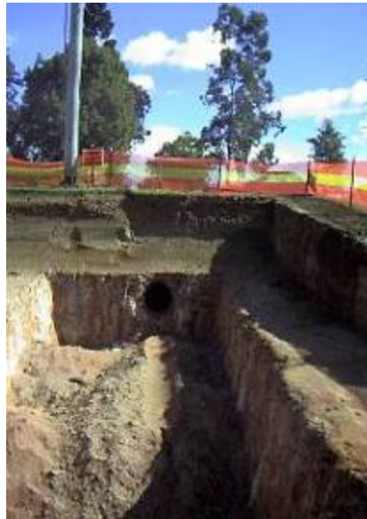
Plate 21: Thrust bore drill hole
