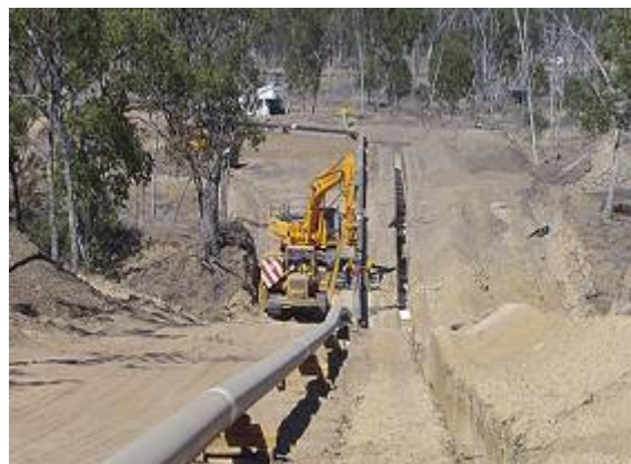
Plate 10: Pipe after welding and coating, before lowering-in
