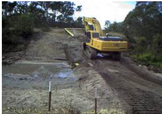
Plate 25: Open cut construction of watercourse crossing
