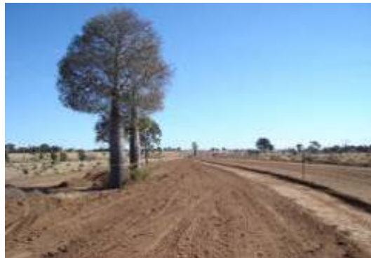
Plate 3: Typical clearing of the ROW and avoidance of sensitive vegetation
