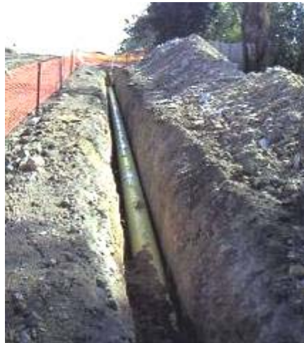
Plate 12: Pipe lowered into trench and spoil backfilled
