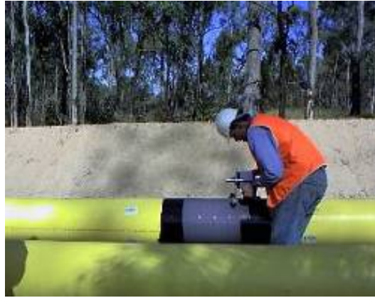
Plate 7: Coating and wrapping of the weld joint
