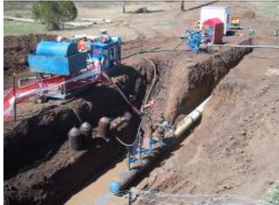
Plate 13: Hydrostatic Testing in progress
