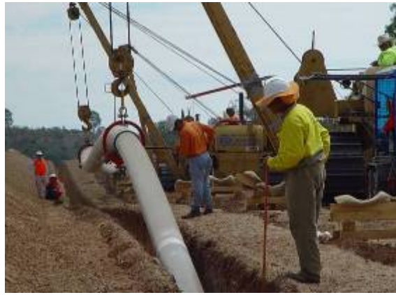
Plate 11: Pipe lowered into trench
