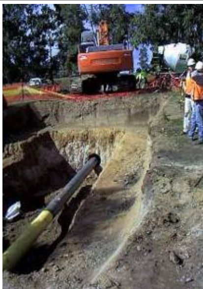
Plate 22: Thrust boring
