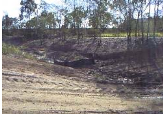
Plate 23: Open cut construction of watercourse crossing
