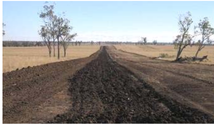
Plate 16: Clean-up of ROW
