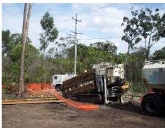
Plate 28: Horizontal directional drilling under a watercourse
