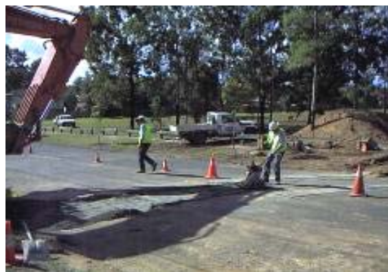
Plate 17: Rehabilitation of ROW across a road
