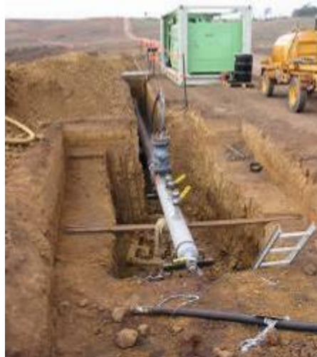
Plate 14: Hydrostatic Testing in progress
